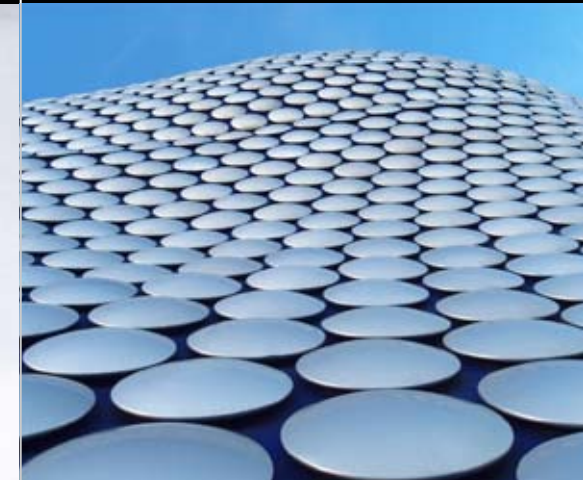
Composite parts bonded to a structure
